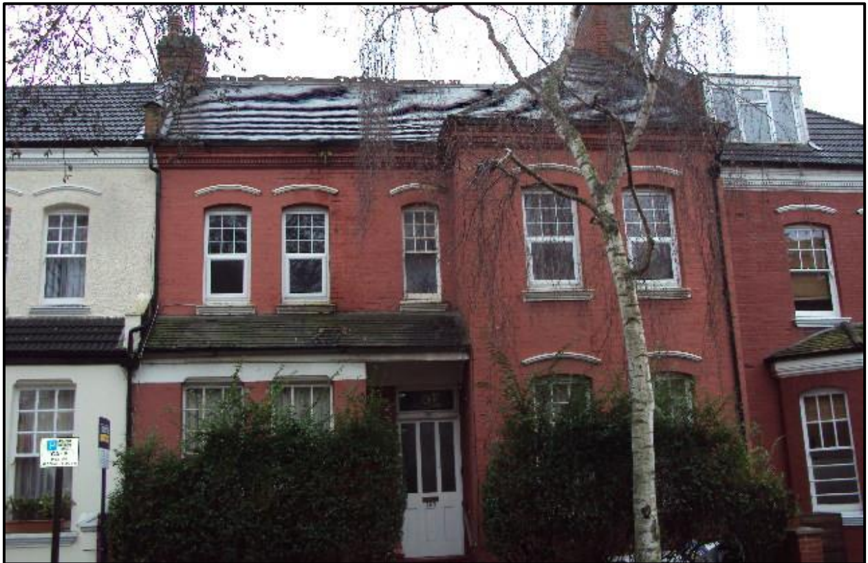
Fig. 1 - Existing view: Front Elevation 163 Sumatra Road
