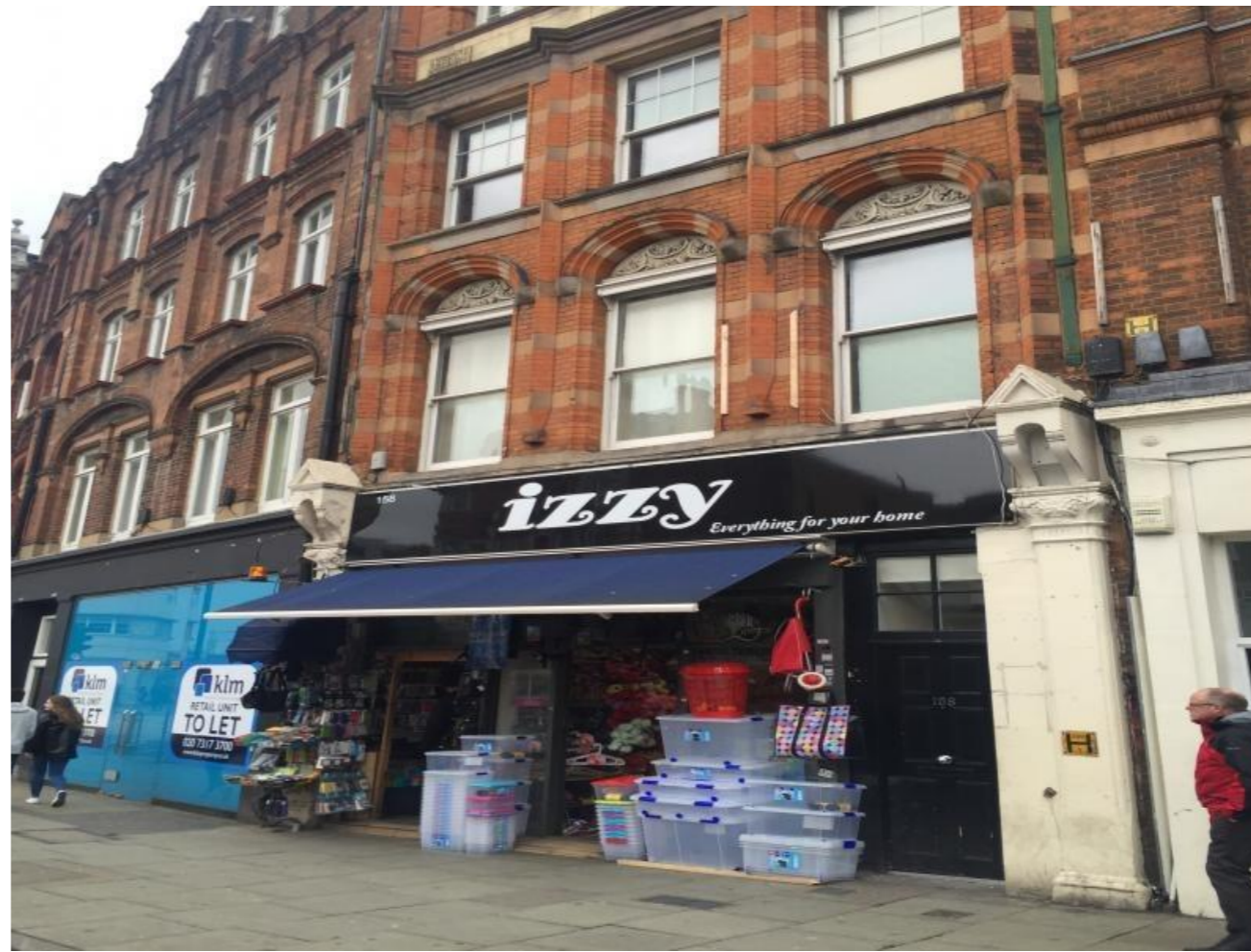
Photo showing the awning opened
