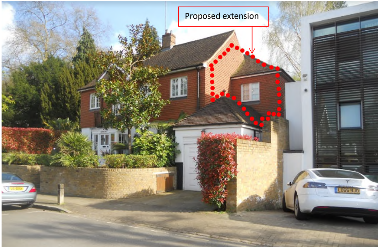
View of the existing building
