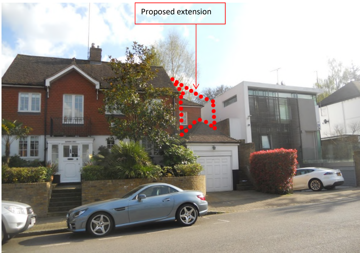
View of the existing building
