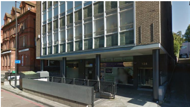
Fig 1 Exterior of 124 Finchley Road
