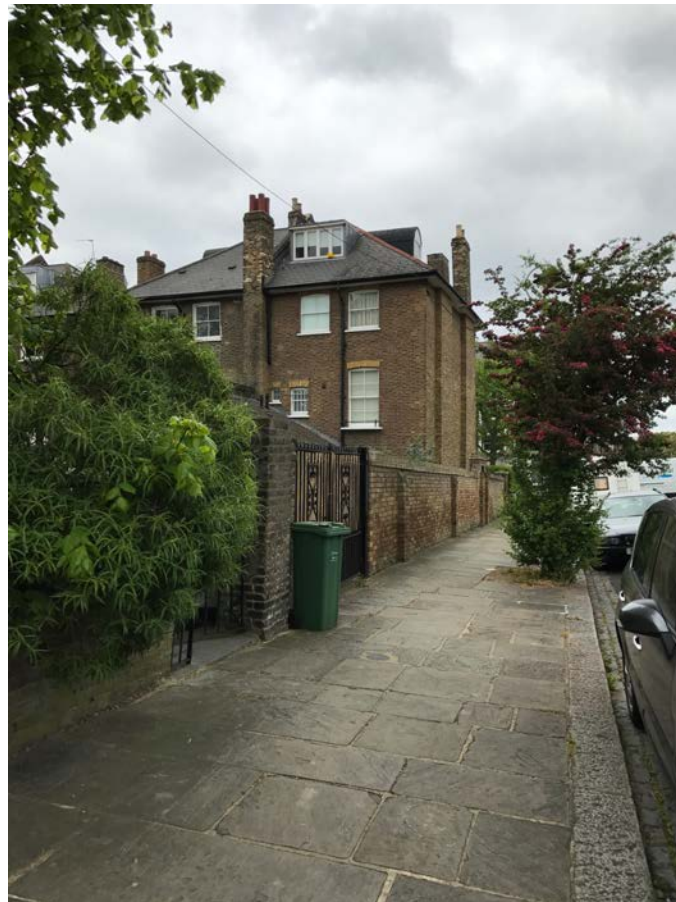
Fig. 3 . Only the very top of the existing roof is visible from the pavement directly adjacent to the boundary wall.
