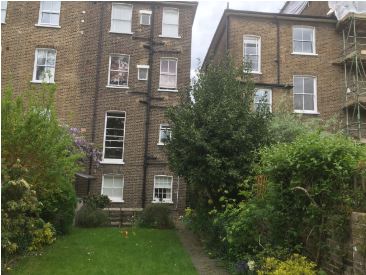
Image 1. Showing the host building in context with no.27.
