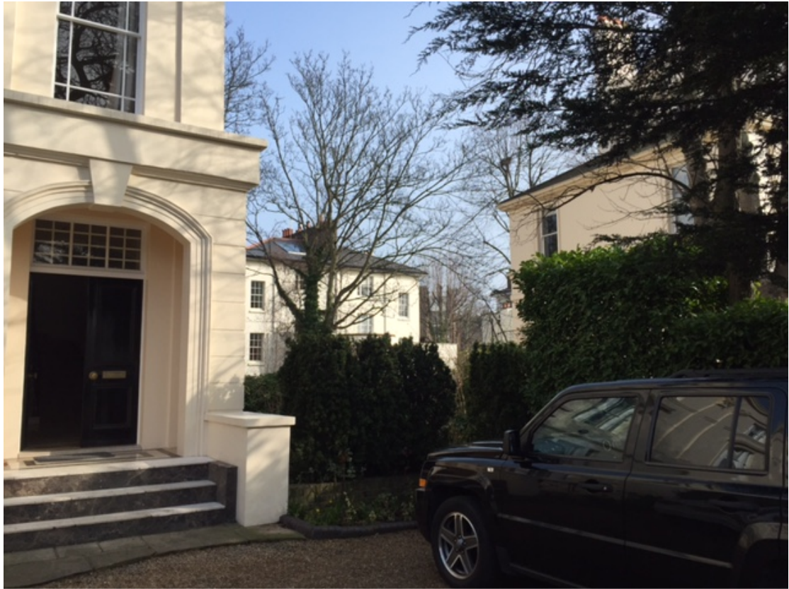
Photo 3: Existing gap between the host building and no.7
