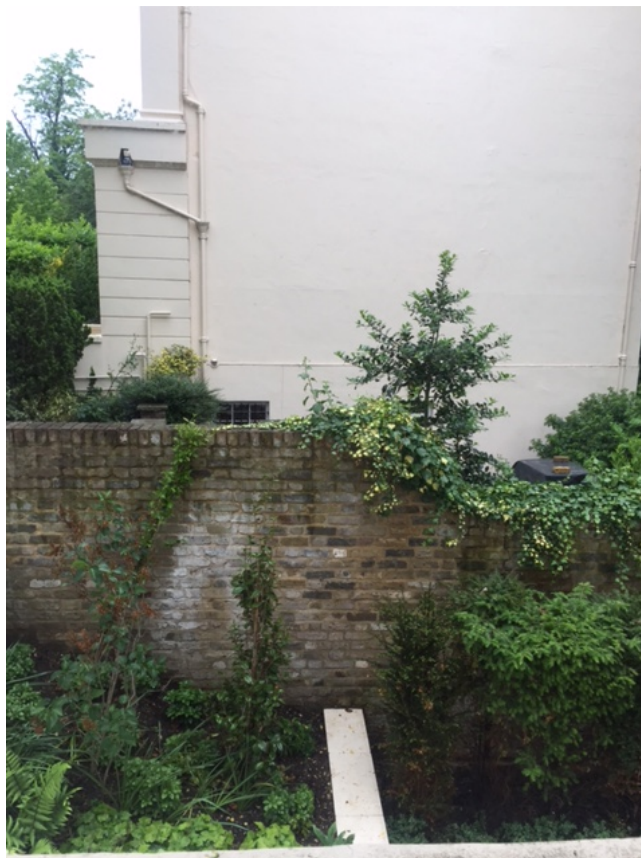
Photo 14: View from first floor of no.7
