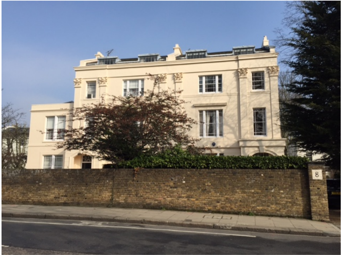
Photo 1: Application building (to the right side) and neighbouring property no.9
