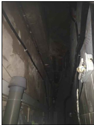
IMG011 SERVICES AT BACK OF PROPOSED RISER CUPBOARD
