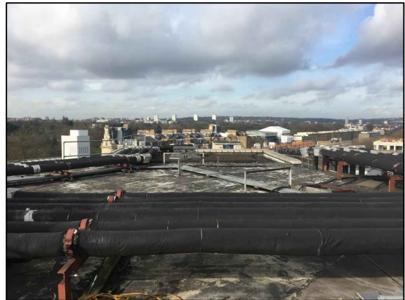
IMG004 PIPEWORK + VIEW ACROSS ROOF
