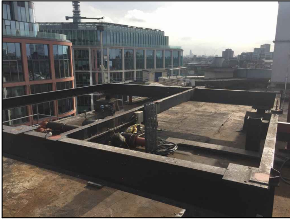
IMG001 EXISTING STEELWORK; PREVIOUS CHILLER
