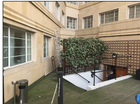
IMG008 POTENTIAL PLANT SPACE BEHIND SCREEN
