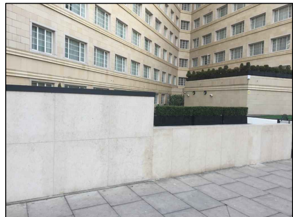
IMG014 REVIEW OF LINES OF SIGHT FROM STREET PERIMETER FOR 'CORNER' OPTION
