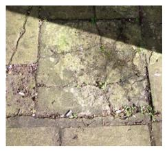
(4) Careful removal of concrete from surface of paviour, assessment of surface condition (Revert to options 1,2 or 3 dependant on condition).
