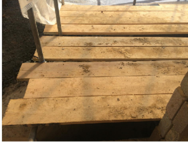
Photograph 1: Example of ground protection using a raised platform on scaffold boards on a scaffold framework
