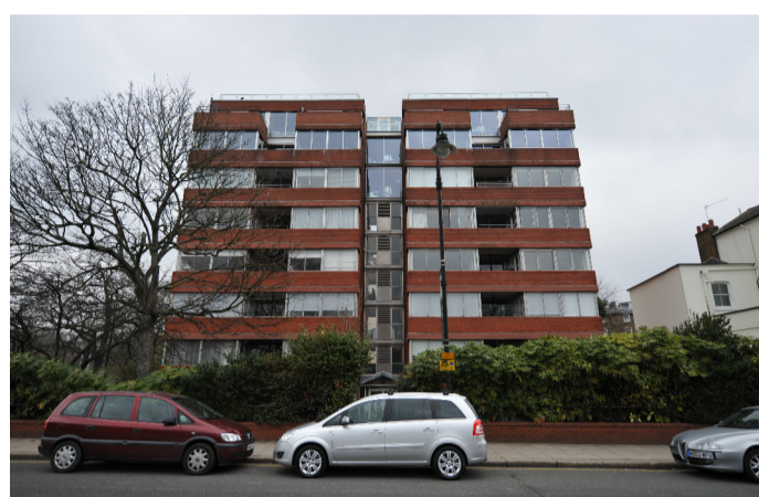
a Prince Albert Rd Facade
