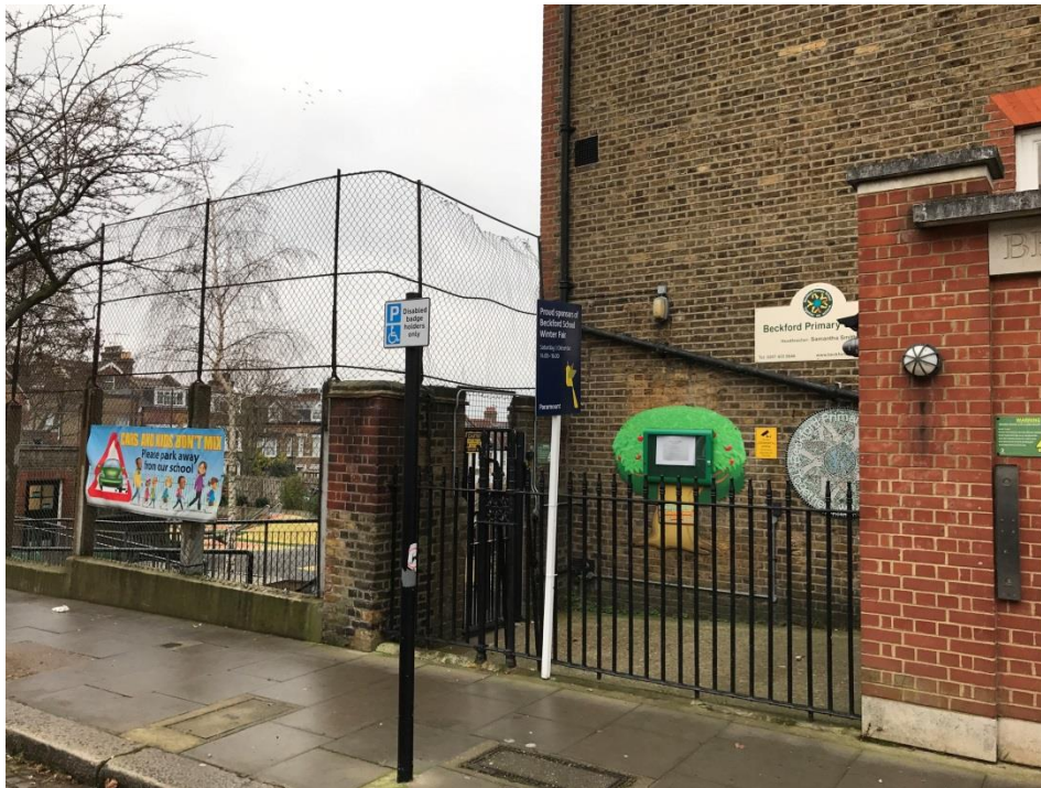
Pic. 1 – Dornfell St (north-west)- brick wall adjacent school's main entrance
