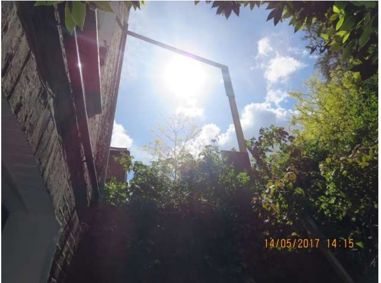
Photo taken from outside our kitchen door. Structure showing how the sun will be obstructed by the proposed extension.
