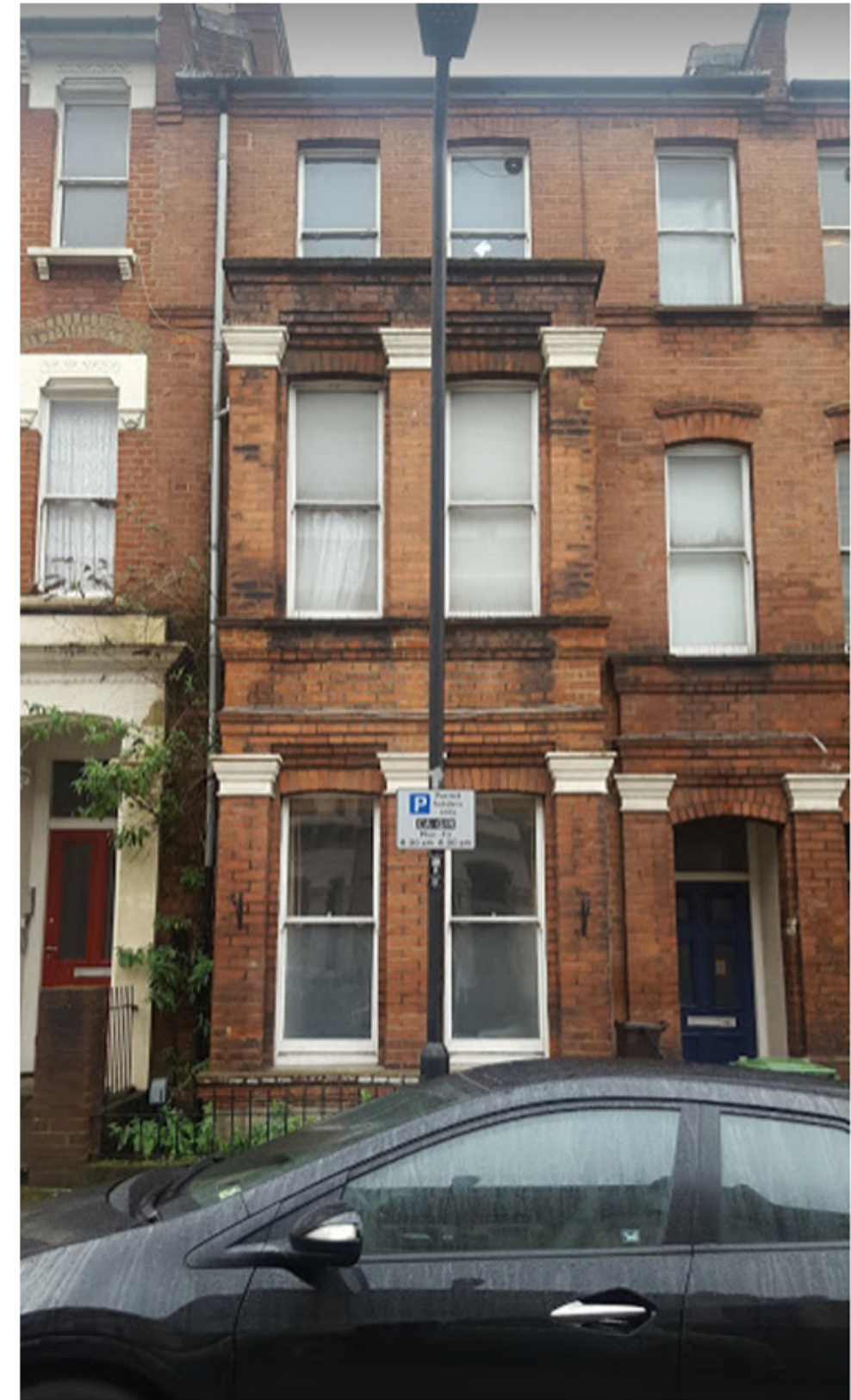
Existing Front elevation photo
