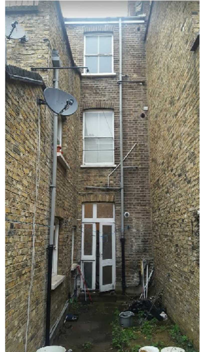
Rear elevation photo
