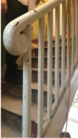
Existing spindles and handrail.
