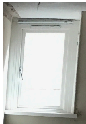
Windows to rear.
