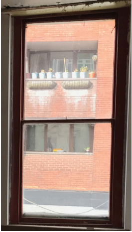
Windows to front facade
