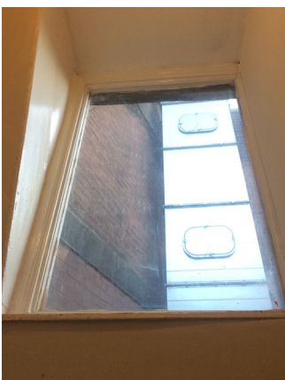
Windows to rear on stairs.
