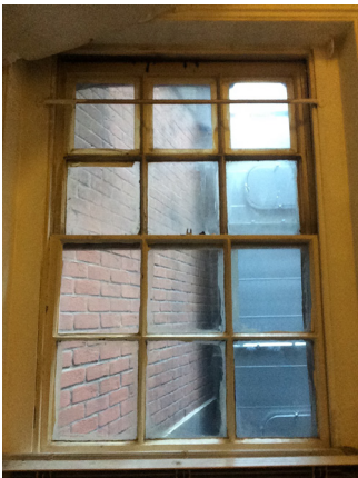
Window to rear on stairs.
