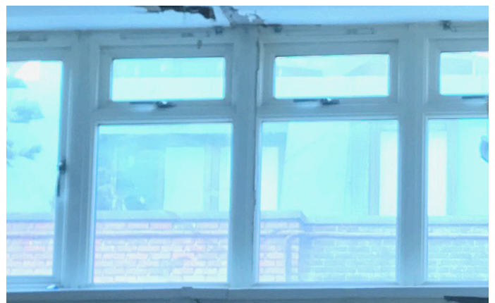
Windows to facade.
