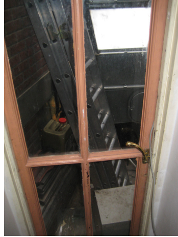
Windows to rear
