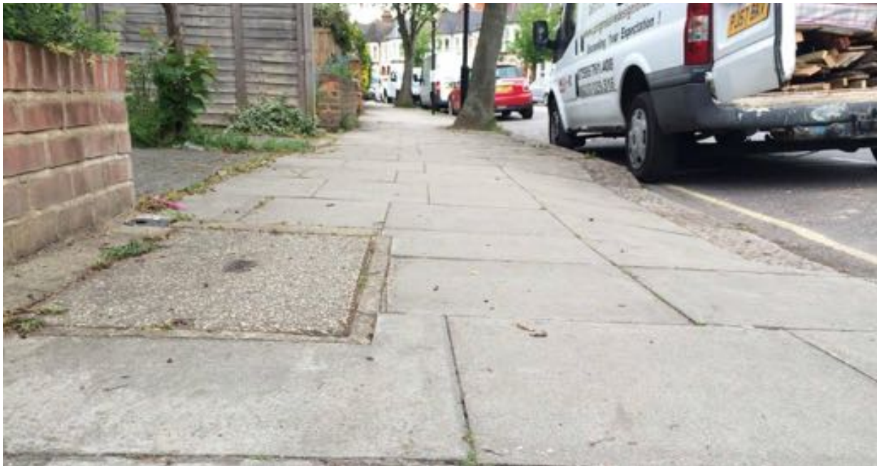
Photo 2: At the front of the house, the footway falls gently towards the Hillfield Road carriageway, away from the property.
