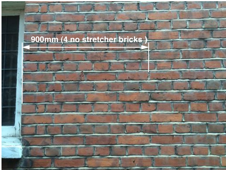
PHOTOGRAPH OF EXISTING FLANK WALL SHOWING THE CLASSIC ENGLISH BOND
