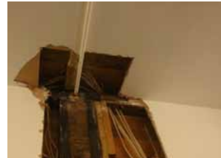
DT1: exposed middle post with steel support
