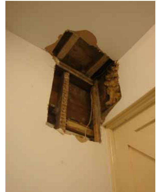
DT2: exposed external wall post
