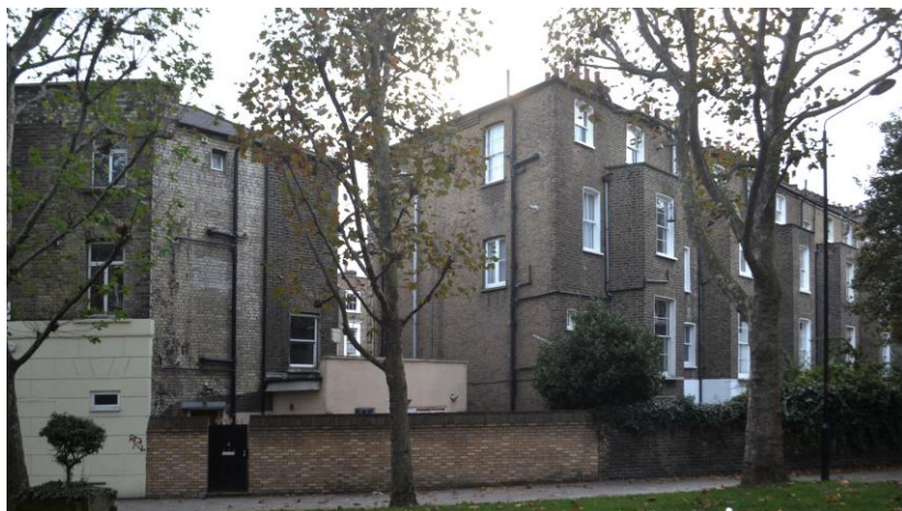
Existing view of the rear of 93 Agar Grove
