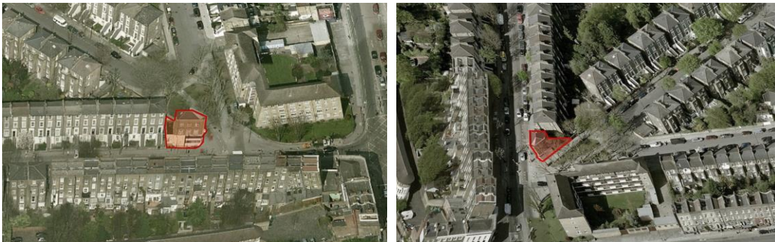
Bird's eye view of site and Surroundings (93 Agar Grove)
