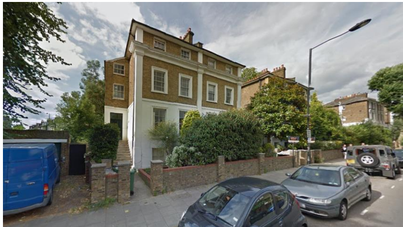
Side staircase example on Agar Grove
