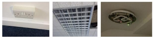
• **Ceilings:** All cornices to be retained and redecorated with white paint. The modern suspended grid ceiling to be strip out and replace with new plasterboard ceiling.
