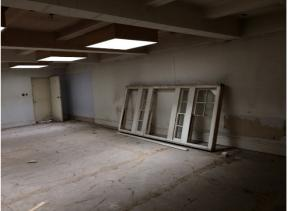
• Internal Walls: All existing walls and mouldings to be retained and redecorate with white paint; all exposed brick work walls to be covered with plasterboard decorated with white paint
