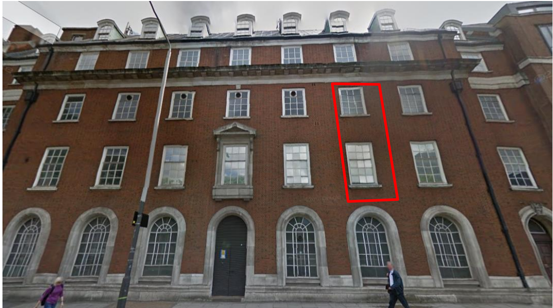
Photo 1- Front Elevation (Red indicating affected windows)
