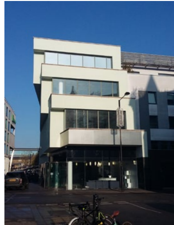
View from Jamestown Road
