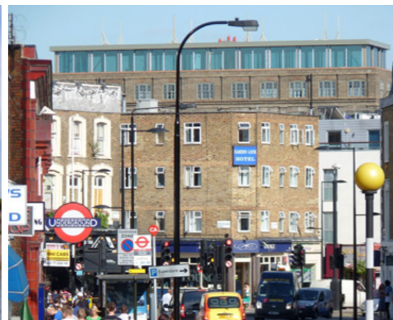
Belmont Street warehouse conversion and roof extension
