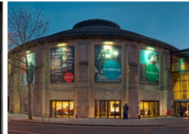
The Roundhouse Refurbishment
