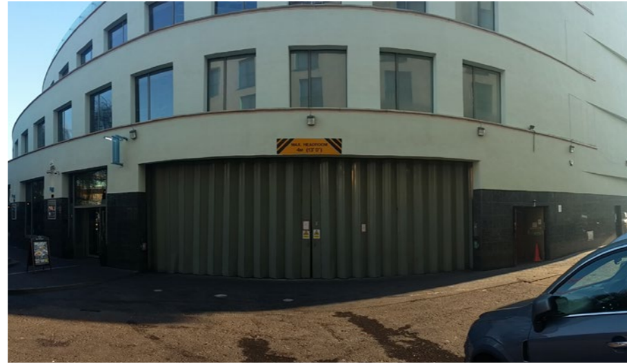
View of existing service yard entrance
