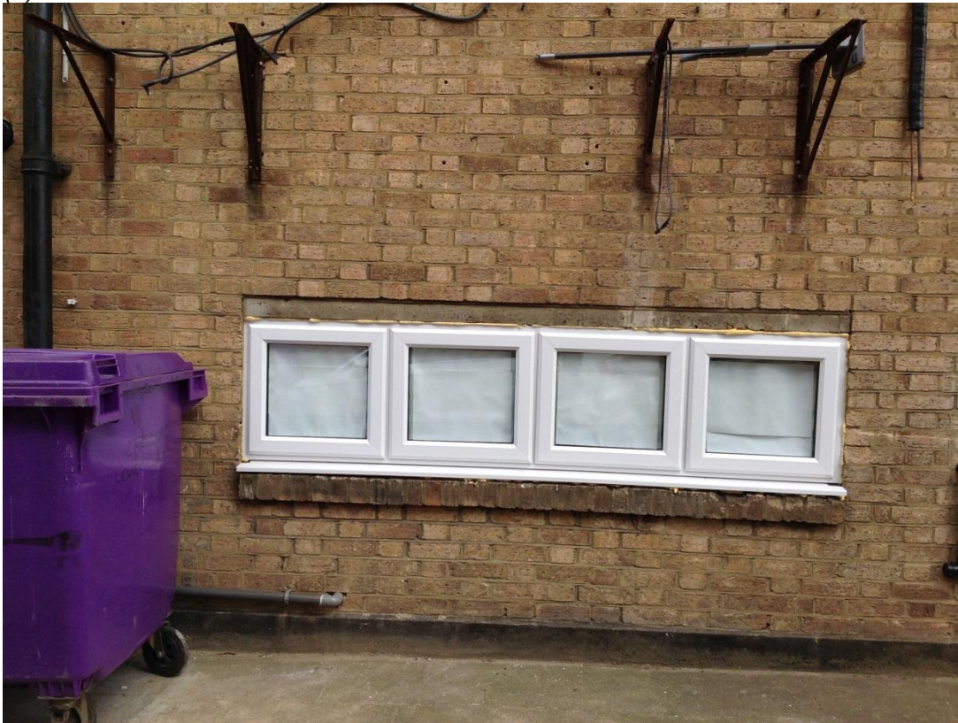
(7) Rear LG floor windows as installed
