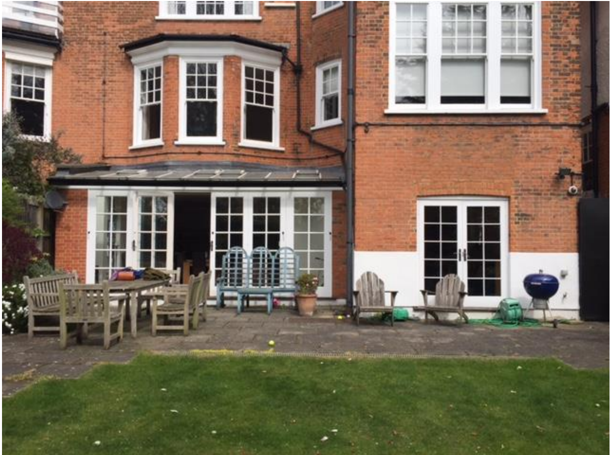
Photo: Existing conservatory and timber doors
