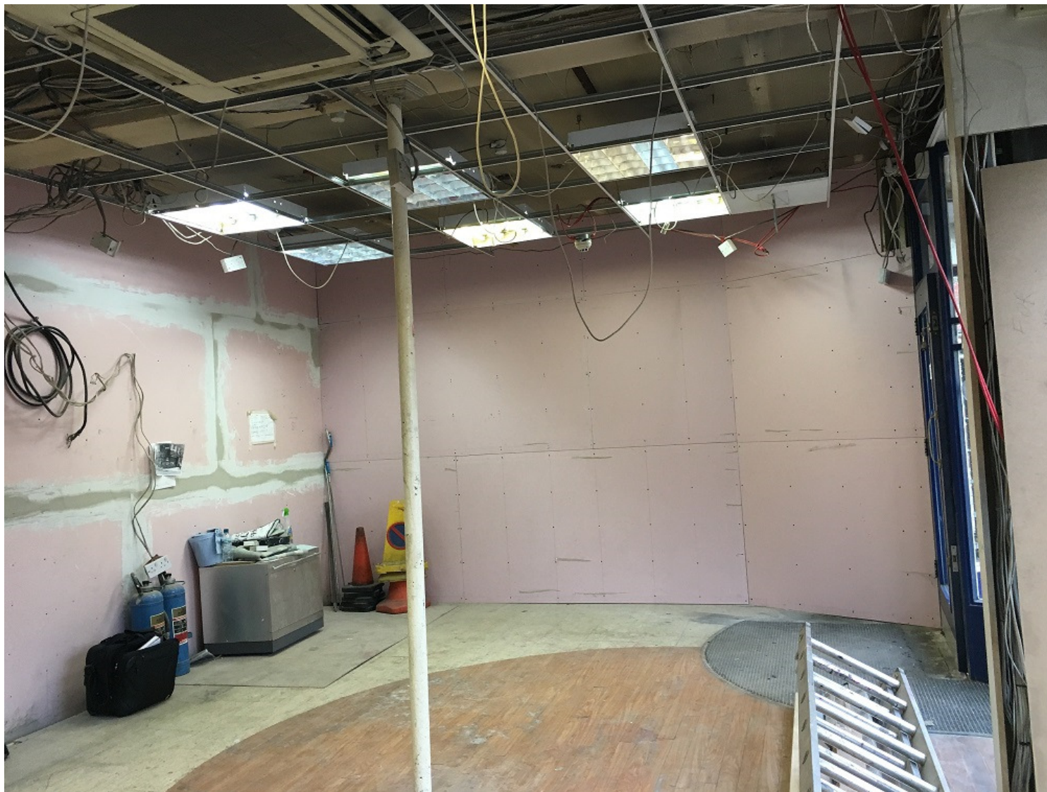
Existing internal site photos
