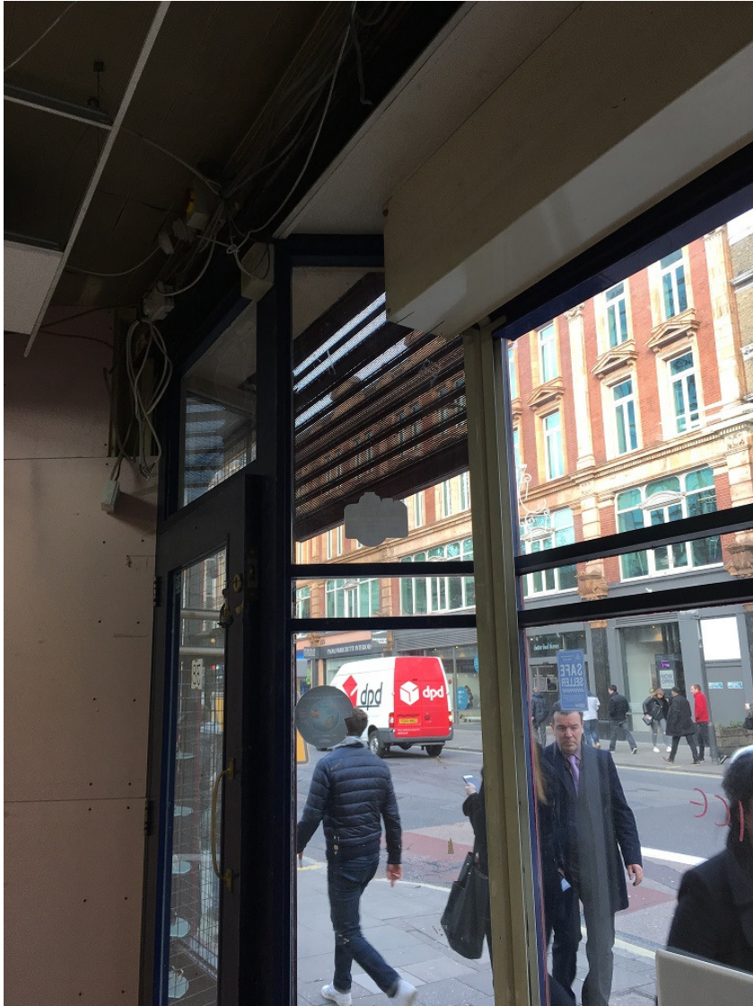
Existing internal site photos
