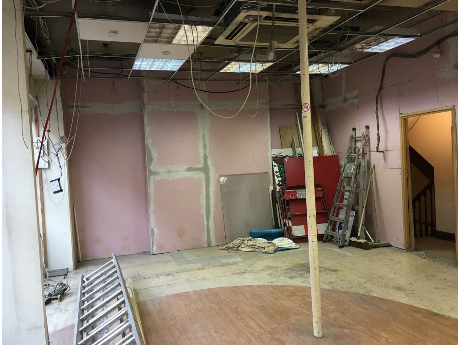
Existing internal site photos
