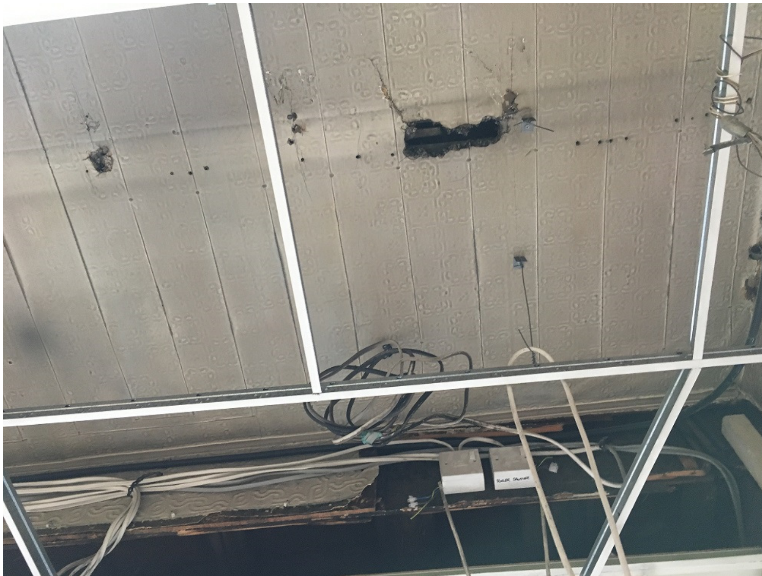
Existing internal site photos
