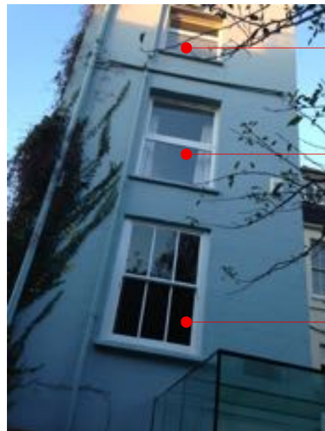
2-W02 SECOND FLOOR REAR WINDOW
