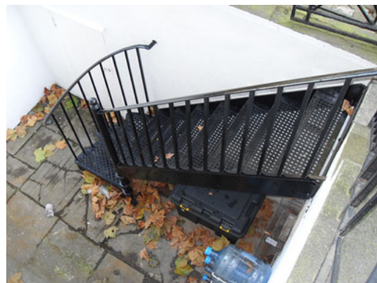
PRECEDENT IMAGE FOR NEW CAST IRON STAIRCASE TO LOWER GROUND FLOOR. OPEN TREAD SQUARE PATTERN GRATED TREADS, 17MM SQUARE BASLUSTRADING AND FLAT CAST IRON HANDRAIL
