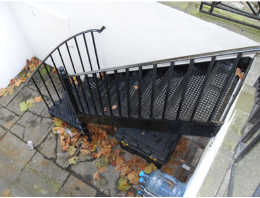
PRECEDENT IMAGE FOR NEW CAST IRON STAIRCASE TO LOWER GROUND FLOOR. OPEN TREAD SQUARE PATTERN GRATED TREADS, 17MM SQUARE BASLUSTRADING AND FLAT CAST IRON HANDRAIL
