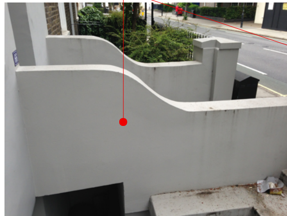
LOW WALL ADJACENT TO LIGHTWELL TO BE REPLACED WITH CAST IRON RAILING TO MATCH NEIGHBOURING PROPERTY
