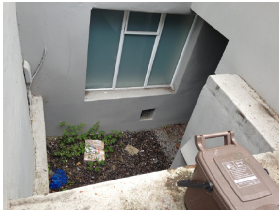
EXISTING IMAGE OF LIGHTWELL WITH EXISTING METAL FRAME WINDOW - WINDOW TO BE REPLACED WITH TIMBER FRAME SASH WINDOW AS PER DRAWING.
