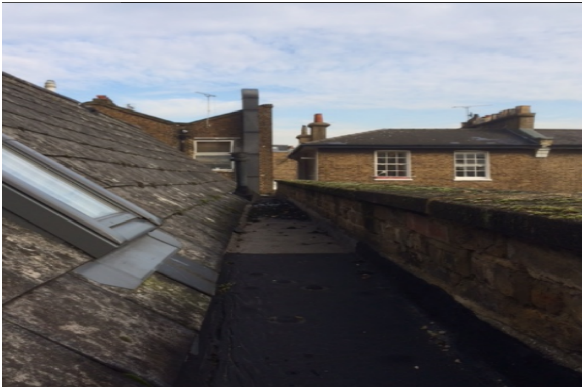
Photograph 2: View towards south-west of the roof slope and proposal area
