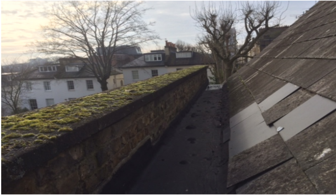
Photograph 3: View towards south-east of the roof slope and proposal area
