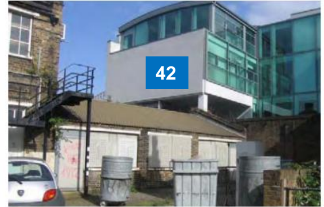
E COURTYARD FACING BUILDING. (DEMOLISHED WITHIN CONSENTED 2012 SCHEME)
