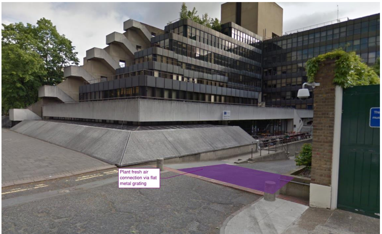
Figure 2 Plant fresh air connection. View from Thornhaugh Street
