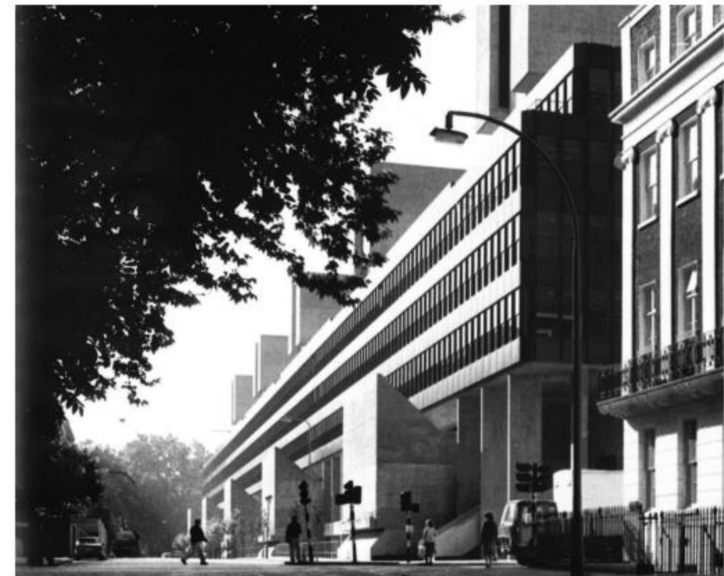
Figure 1—1: UCL IoE building (Hawkins Brown image)
