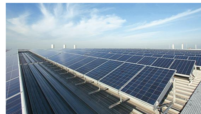
Typical Roof Mounted Solar PV Array
