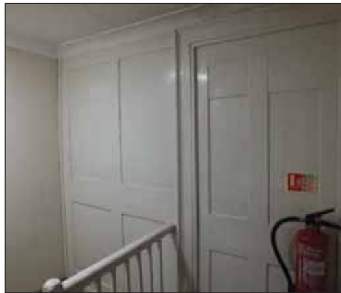
Photo 7: Wooden panelling and blocked door in No. 109 third floor / attic level, hallway
