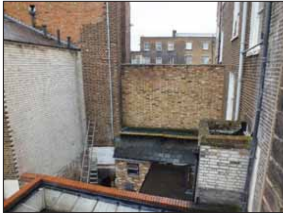
Photo 10: View towards area to be developed from No. 109, looking north-east
