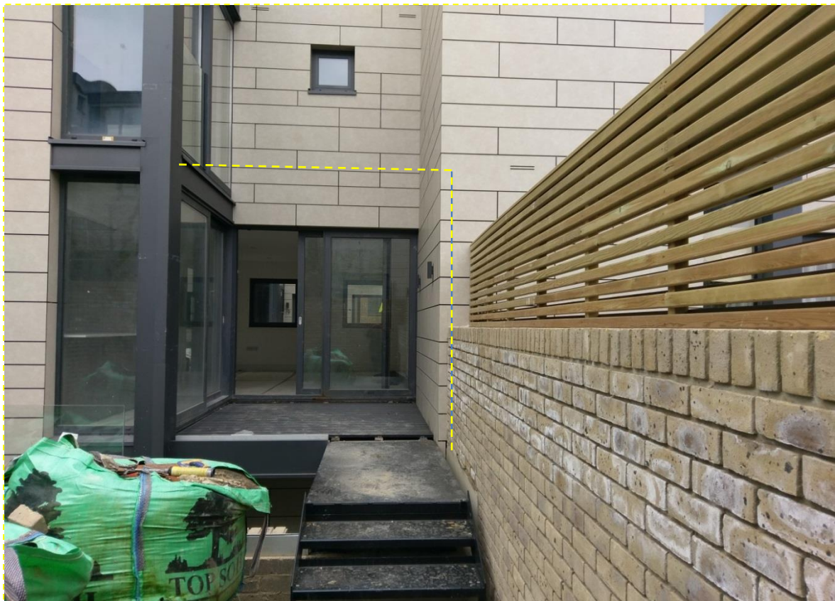
Photo.3 View back towards No.10 indicating area of infill extension.
