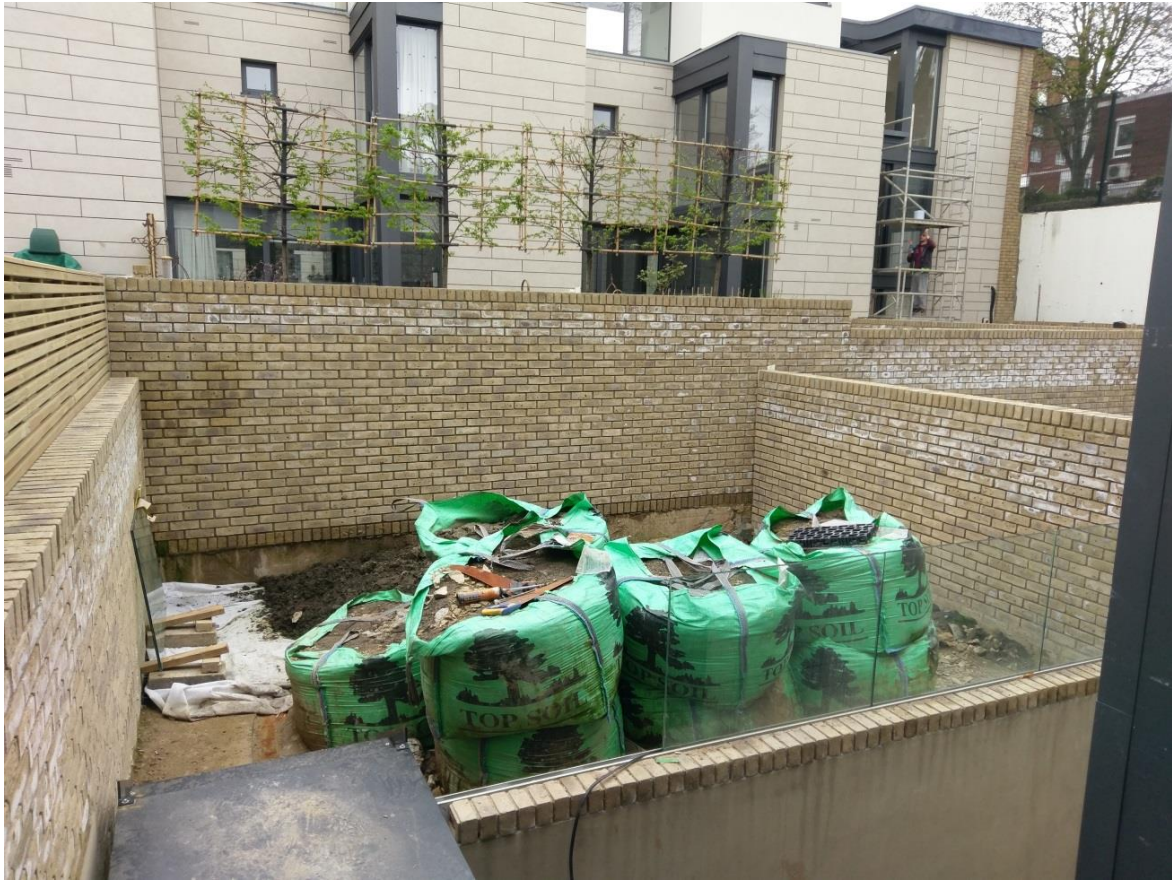
Photo.2 View from proposed line of extension looking west
