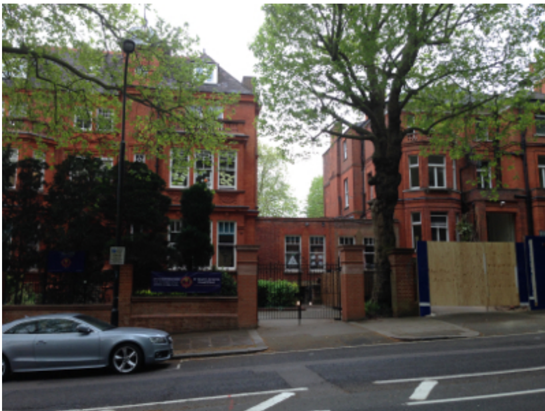
Photograph showing both 47 and 49 Fitzjohn's Avenue and the link between both buildings.
