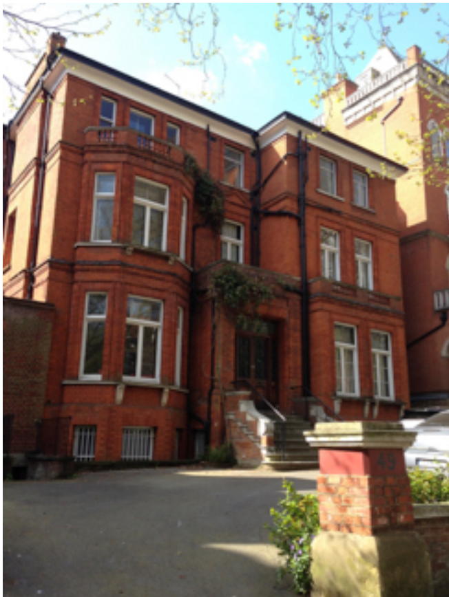
Front Elevation of 49 Fitzjohn's Avenue
