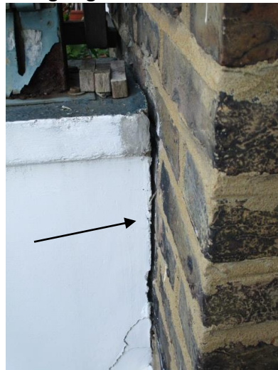
Separation at rear addition junction viewed from upper flat roof terrace
