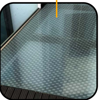
Entrance Walkway Floor Frosted & Fritted Dotted Glass
