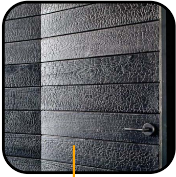
Right Side Cladding and Service Door: Shou-Sugi-Ban
