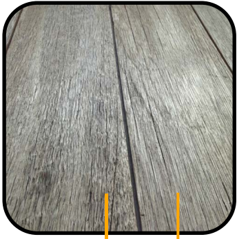
Left Side Cladding & Main Entrance Door: Oak Panels (shown after ageing)
