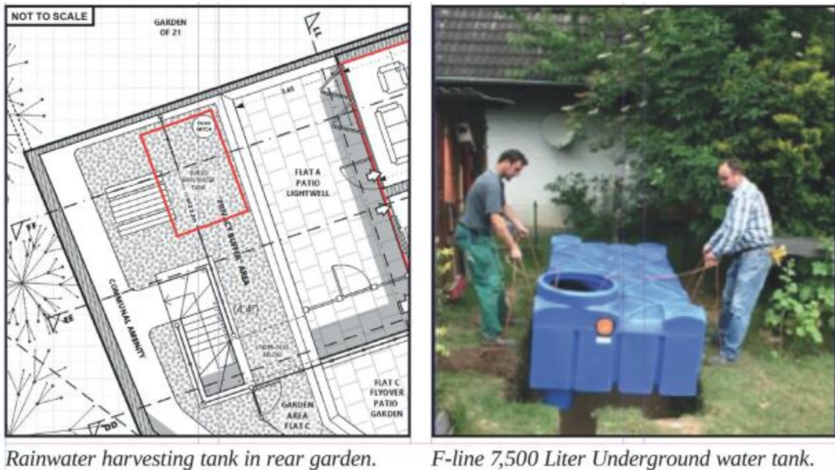
Figure 16: An F-line 7,500 litre underground garden water harvesting system tank will be installed on site, accessible for maintenance, buried in the rear communal garden.
