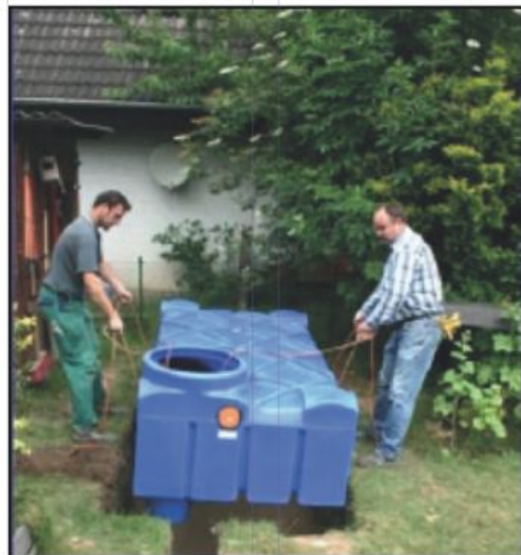
F-line 7,500 Liter Underground water tank.
