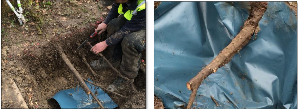
Fig. 2 Root exposure and treatment – manual working, sharp tools and clean cuts
