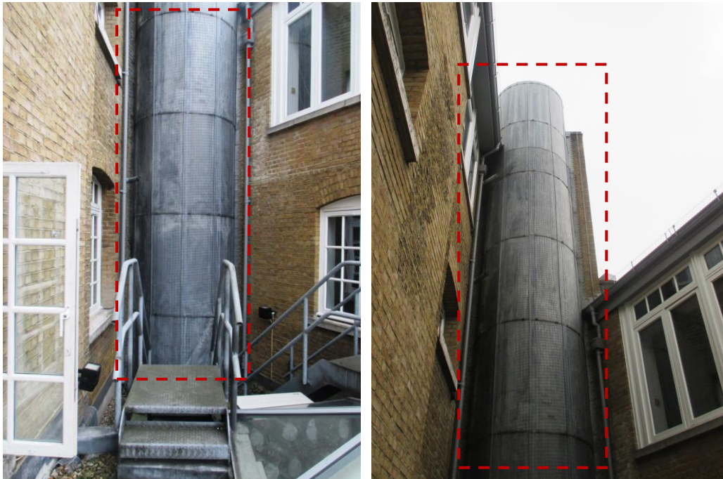
Existing Vertical Shaft to the Rear of Thomas Neals
