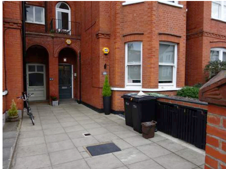
View towards front doors of 60 and 62 Crediton Hill
