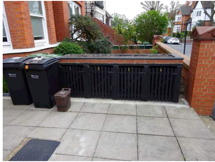
Existing Bin store in garden of 60 Crediton Hill
