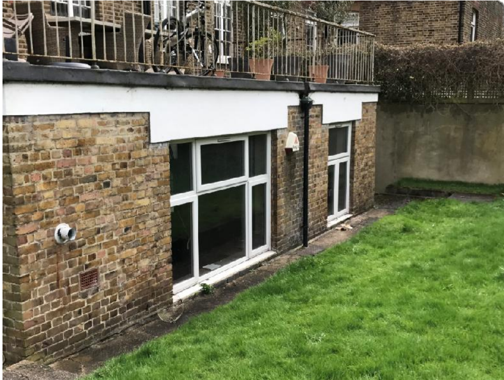
Photograph 02 - Rear elevation - indicating the UPVC windows to be removed.
