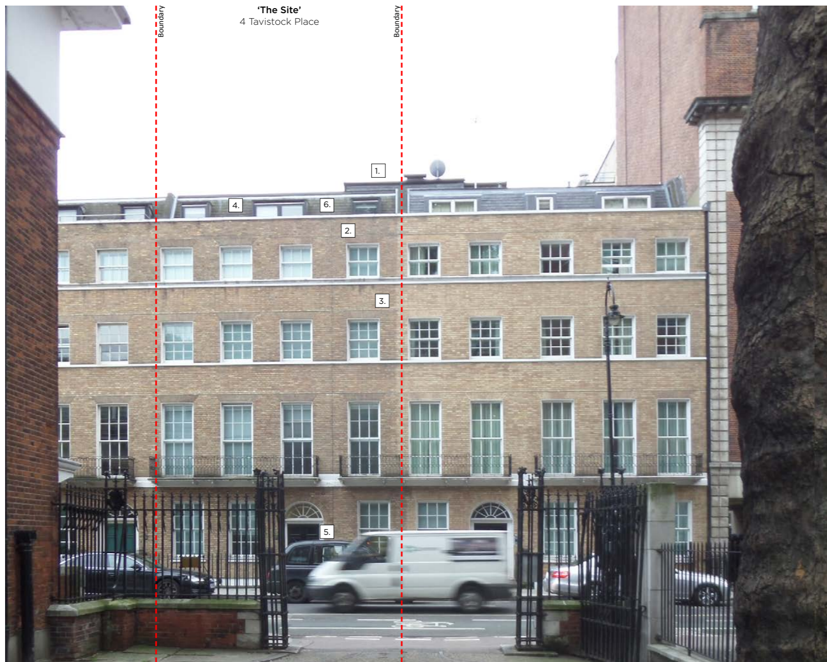
No.2, 4 & 6 Tavistock Place As seen from Mary Ward House. The portion of the roof level shown here cannot be seen from the public highway (Tavistock Place).
