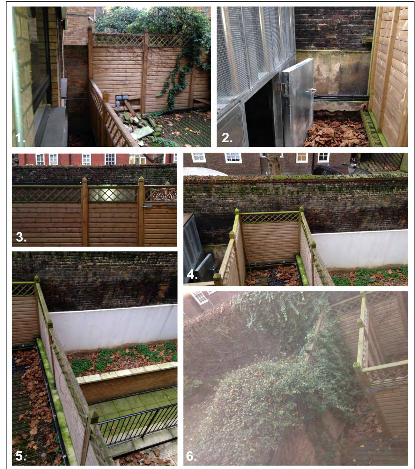
Figure 4: Photographs Indicating the Rear Boundary Conditions
