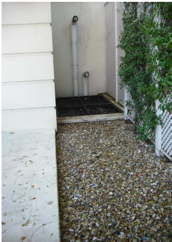
Fig 3 – Rear boundary wall to Number 48
