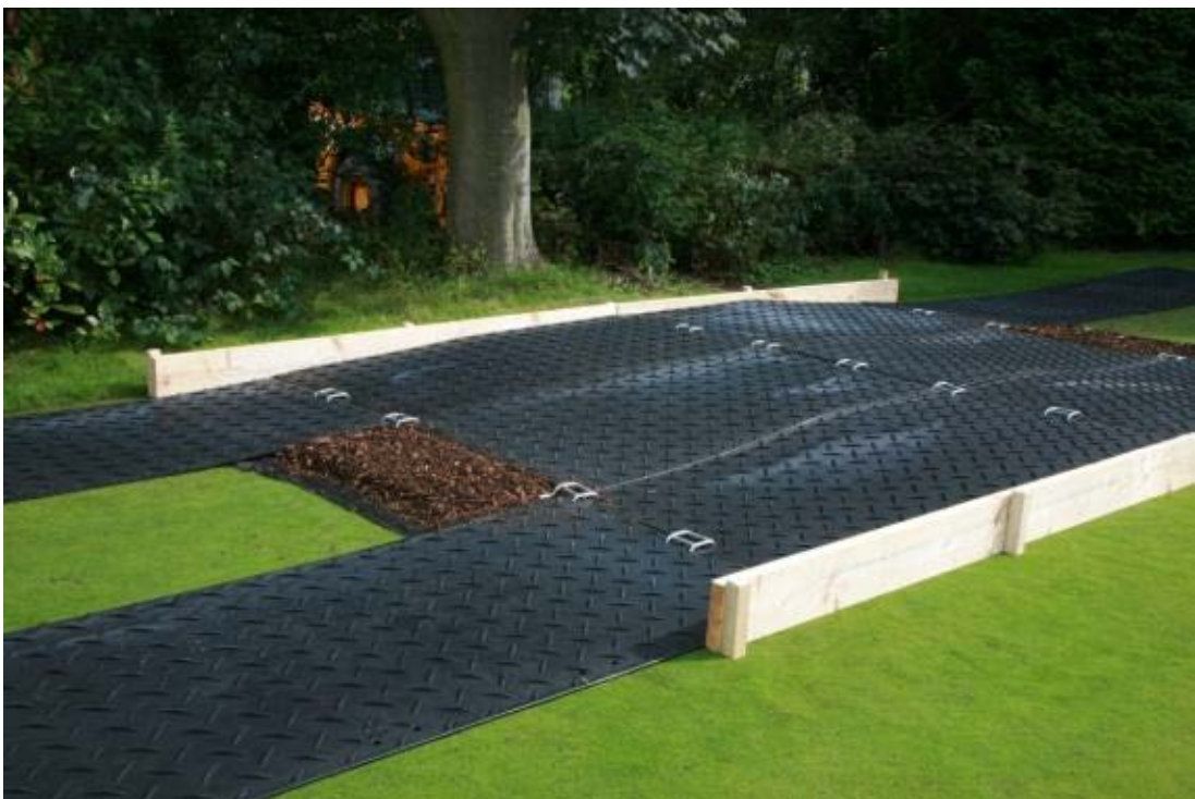
Photo 2: Ground-Guards, installed using a geotextile membrane, ground panels, 150mm deep woodchip and ground panels on top and held in place with edge rails. Please refer to www.ground-guards.co.uk/ for more details.
