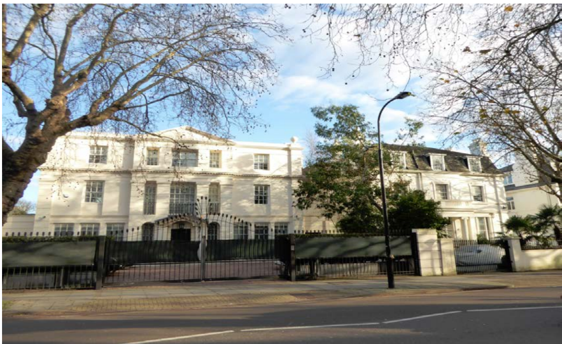
Photo 2 (RM 1.12.15) View of the site, aspect looking north
