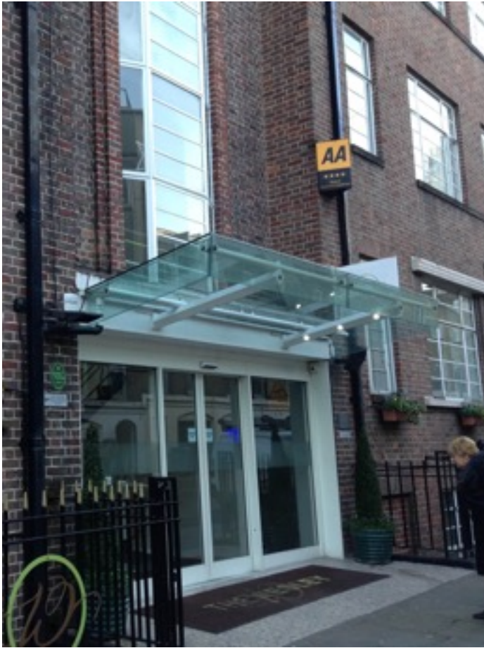
Existing entrance canopy, signboards, and plaques to be removed ( 16, 17 ).
