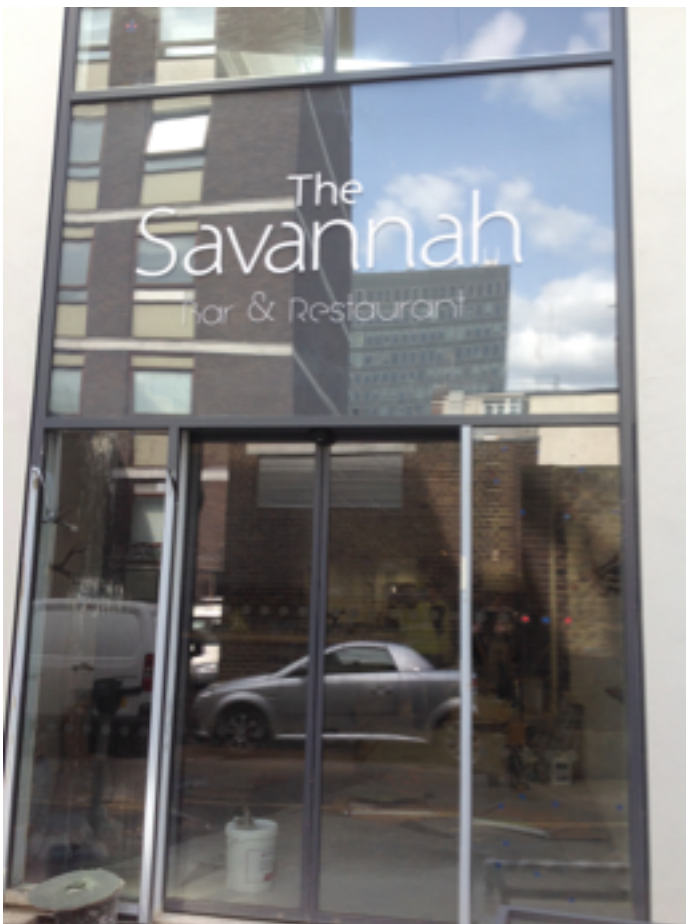
Unconsented flat fascia signage to Regnart Buildings elevation (15) .
