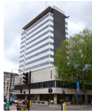
Tall buildings in close proximity
