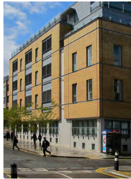
Large developments, Lambs Conduit Street
