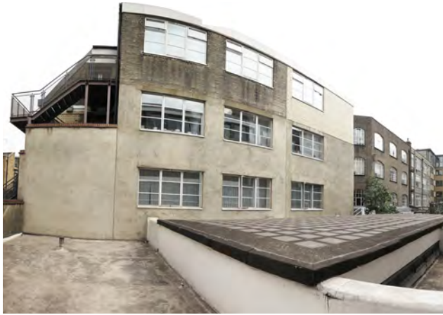
23-29 Emerald Street, rear elevation. Offices overlooking the roof of Bedford House gymnasium.
