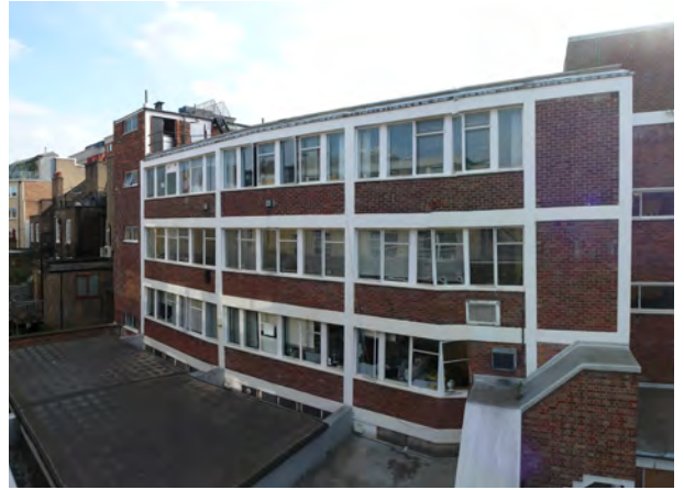
Rapier House, rear elevation. Offices overlooking the roof of Bedford House gymnasium.
