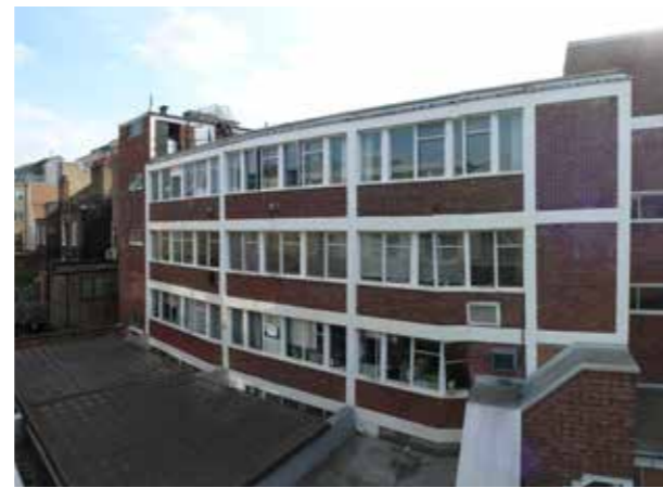
Rapier House, rear elevation. Offices overlooking the roof of Bedford House gymnasium
