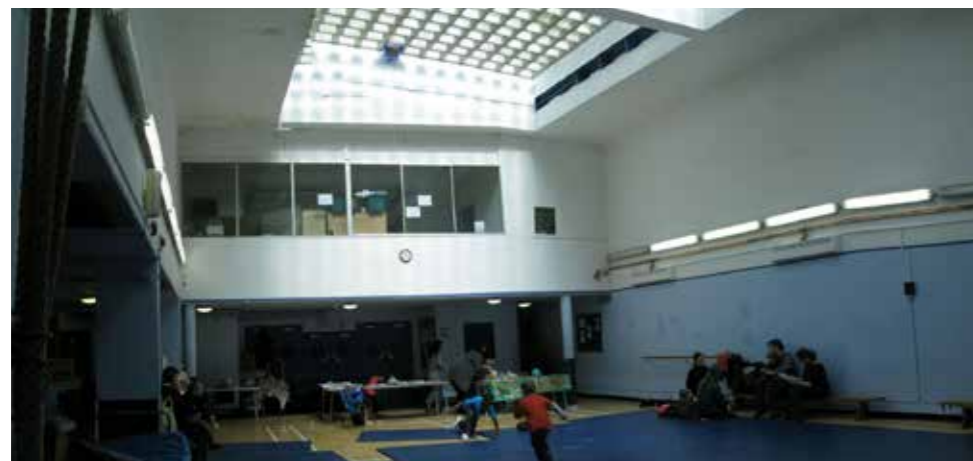
Poor environmental performance - poorly ventilated and lit. Uninsulated
