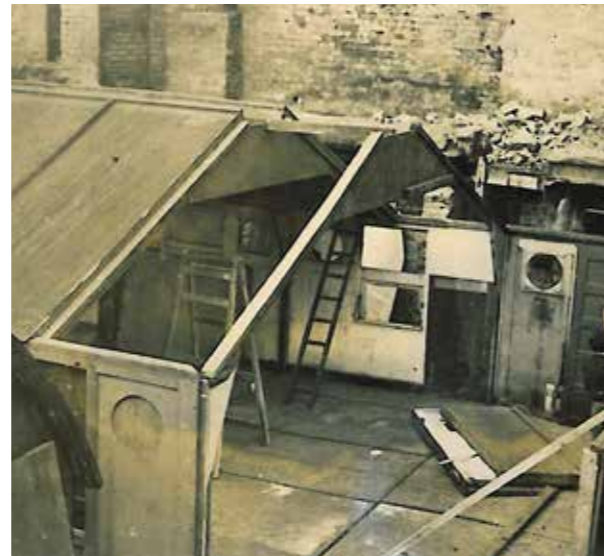
The two huts under construction, they were erected with the efforts of 'Old Bedfordians', ex-Bedford School Boys
