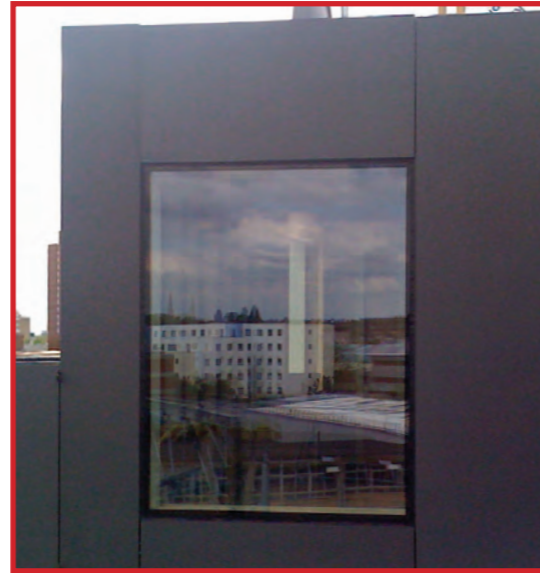
Flush glazed, powder coated aluminium windows with slim sight lines to match existing
